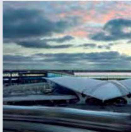
JetBlue, Terminal 5, JFK New York, New York, USA
