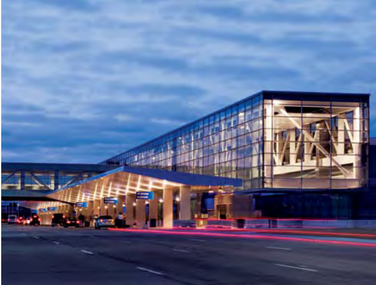
Detroit Metropolitan Wayne County Airport, North Terminal Romulus, Michigan, USA
